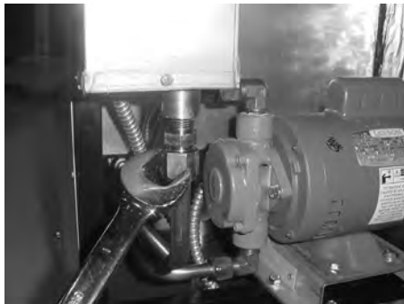
Condensation Box Fitting Step 1
